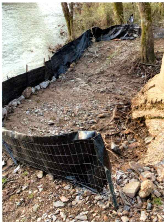
MH 1748 After cleanup
