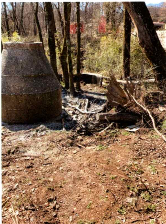
MH 1748 After cleanup
