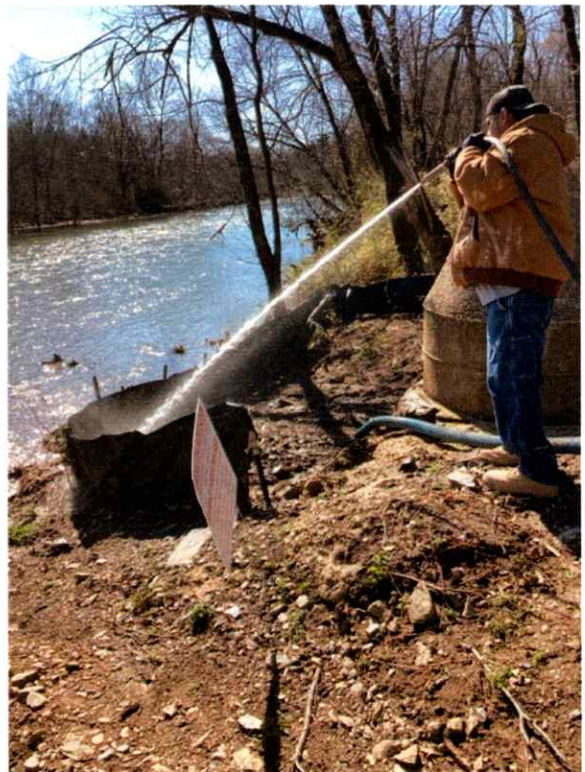
MH 1748 During cleanup
