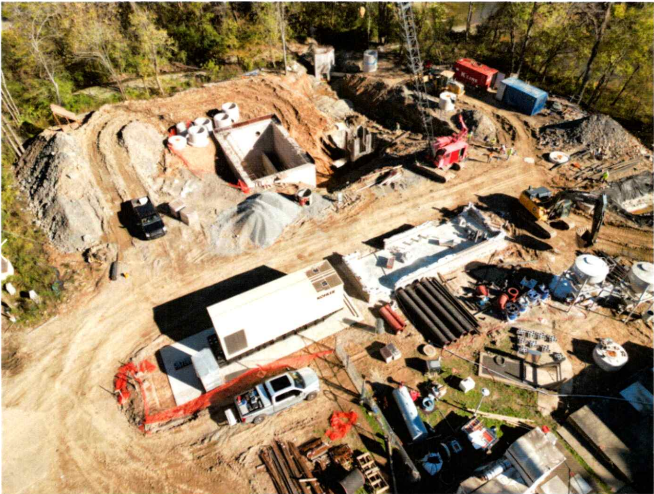
Construction Progress Images for Gulpha Pump Station
